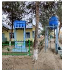
Overhead Water Tank
