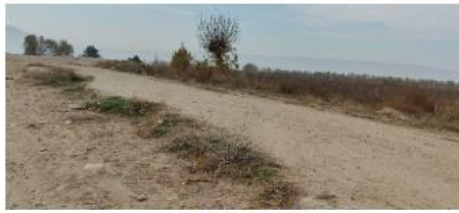
No shoulder/footpath on the road
