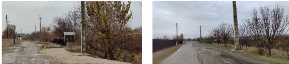
Existing old and new poles are on the roadside
