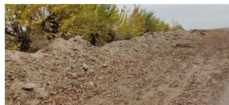
Loose earthen soil on the roadside
