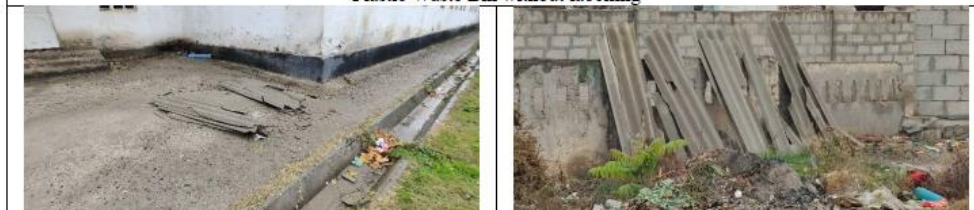
ACM left over at the school campus
