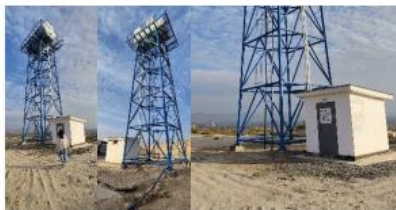
Overhead tank, transmission Pipe and RO facility (in the small room)
