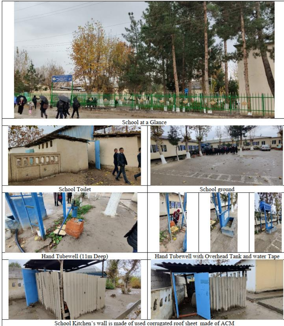
School Kitchen's wall is made of used corrugated roof sheet made of ACM
