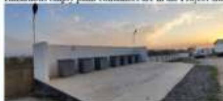
Existing waste storage area of the project site
