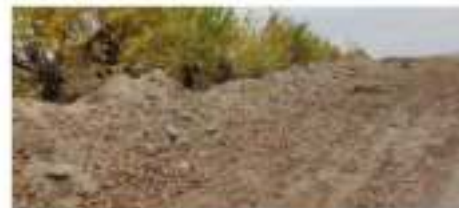
Loose earthen soil on the roadside
