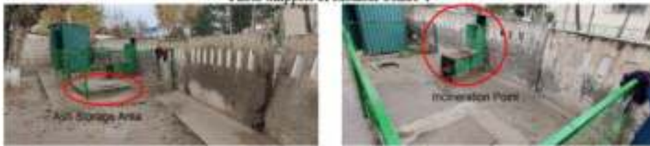
Waste storage and incineration (Local) point
