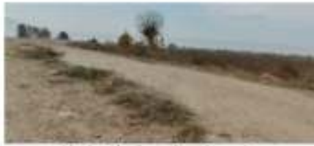
No shoulder/footpath on the road
