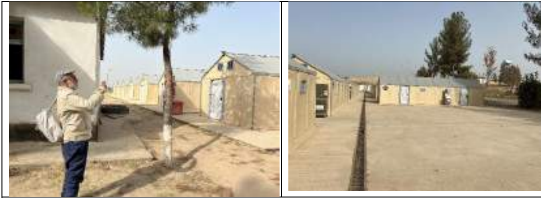
The existing Shelter at the CESED site
