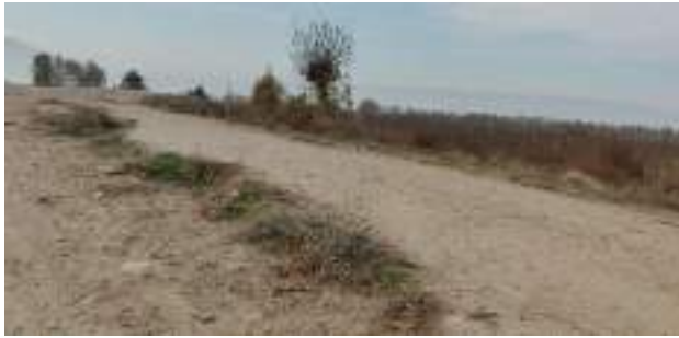
No shoulder/footpath on the road
