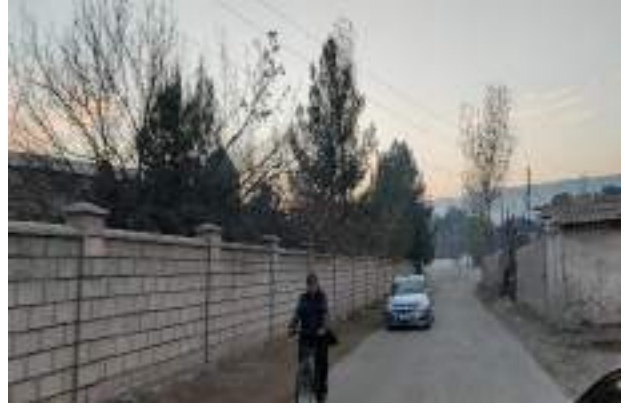
Access road in good condition
